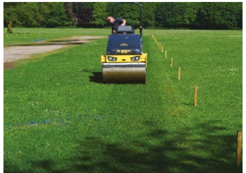
Roll area to push grid into grass
