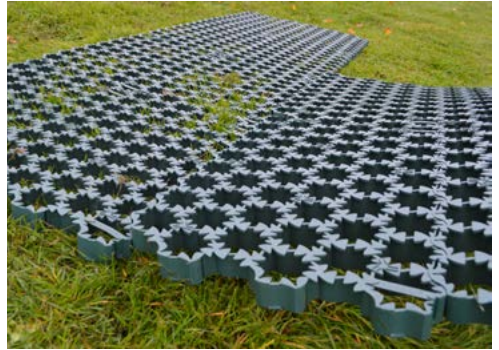
Clip next paver into previous paver
